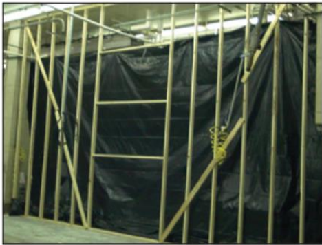
Temporary barriers can protect the production environment from aerosols and traffic that may carry Listeria exposed during construction.
