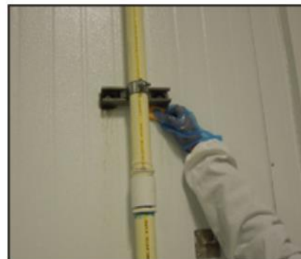
Condensation on walls, ceilings and behind pipes and conduit has been shown to promote Listeria establishment in the facility. Dripping to a concrete berm at the floor, especially if poorly grouted and sealed, can lead to intrusion of insulation and become a long-term reservoir for periodic contamination.
